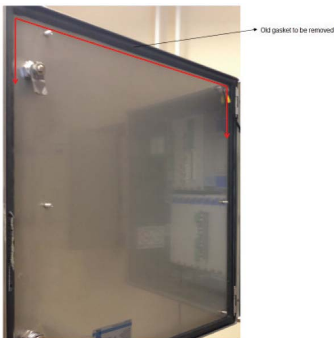
Figure 1. Old gasket to be removed
