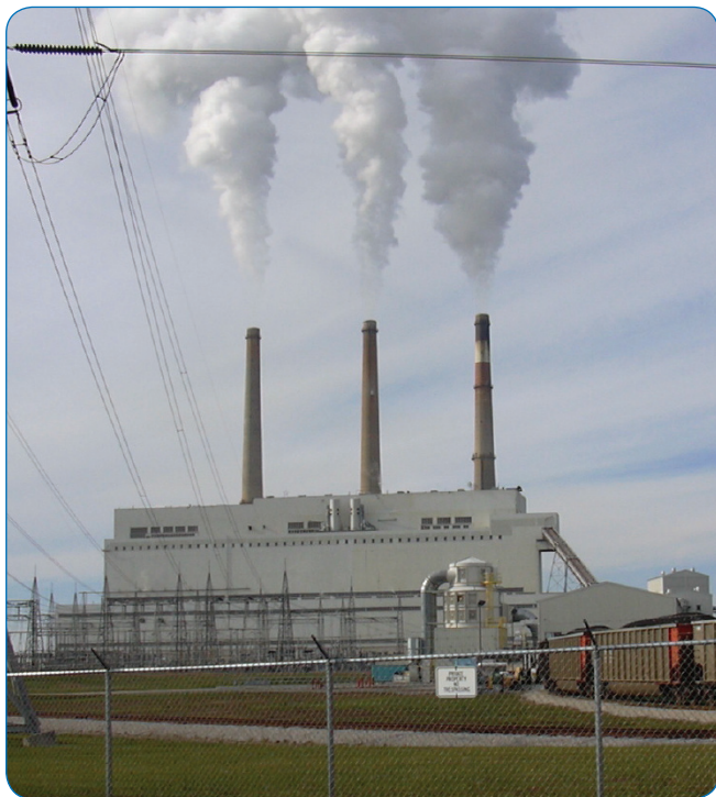
Figure 1. Dynegy's Baldwin Energy Complex.
