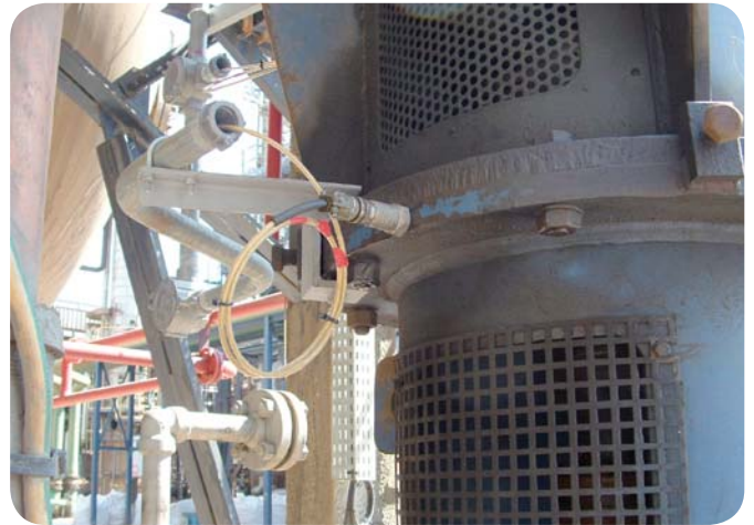
CMSS 786A-IS Industrial Accelerometers – radial direction, stud mounted.
