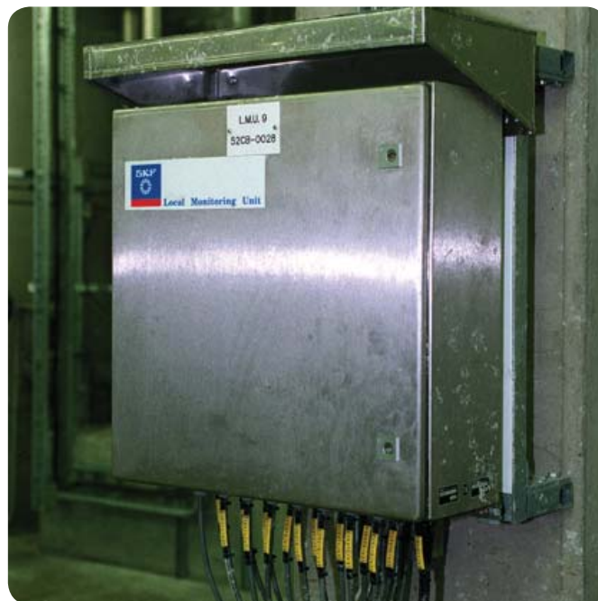
Fig. 2. SKF Multilog Local Monitoring Unit (LMU).
