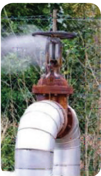
Figure 4. Valve leak.
