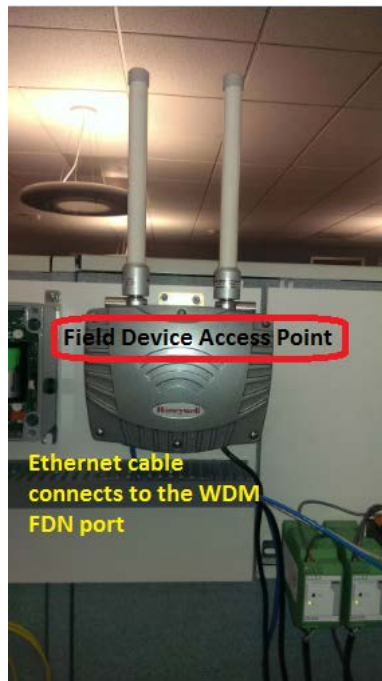
Figure 4 - 1. Connect the FDAP to the WDM FDN port.
