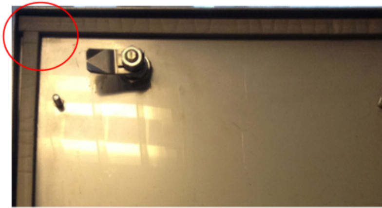
Figure 5-3: Example of homogenous gasket
