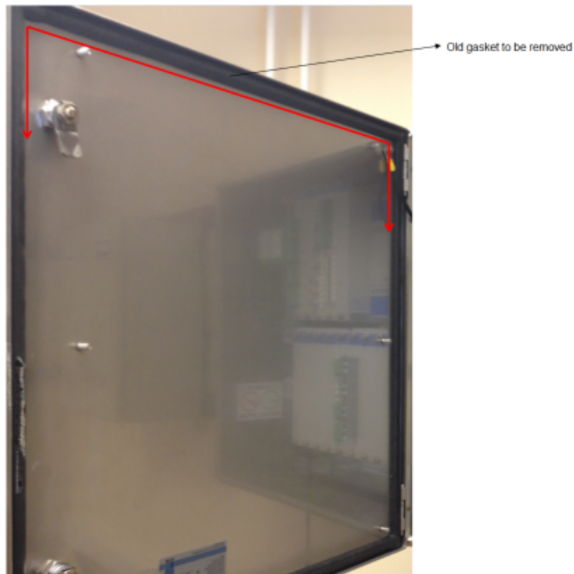
Figure 5-2: Old gasket to be removed
